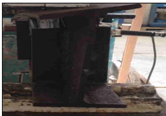
Figure 8: Local buckling of the steel web.
