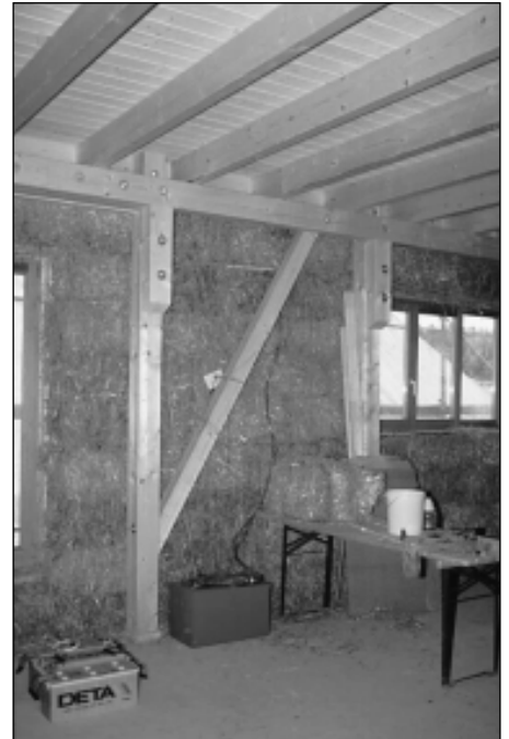
Fig. 1: Medium range measuring (temperature and rel. humidity) in a straw bale wall (wood framing) in a house in Junkershausen
