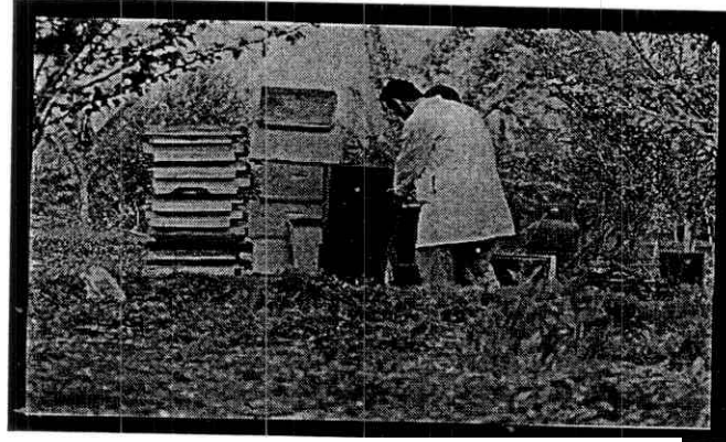
( Figure 78; Consideration to presence of 30cm. space allowed between surface of the wood and the blowtorch ).
